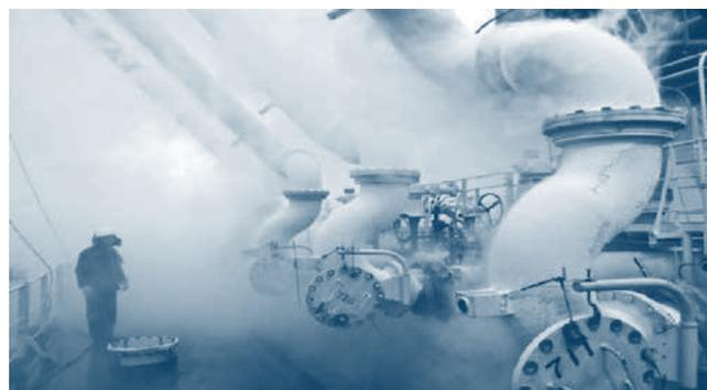
**Figure 6** Vapour cloud resulting from condensing LNG. (Source: magazine.sfpe.org).
